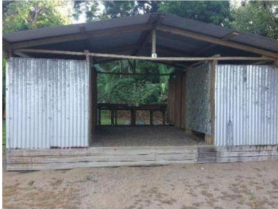
Bathrooms (right) and toilettes (left)
